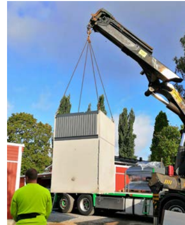
Figure 1. Correct lifting method
