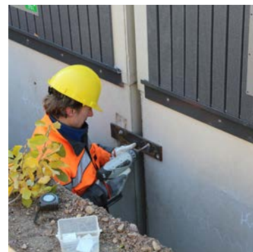
Figure 6. Tying the container bodies together
