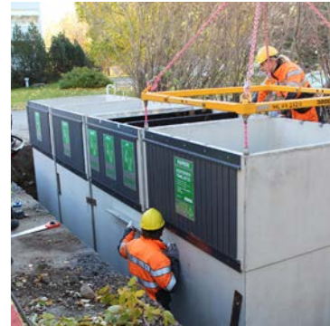
Figure 5. Checking the straightness
